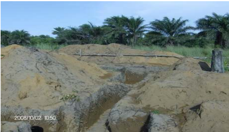
EXCAVATION OF COLUMN & WALL FOOTING TRENCHES.
