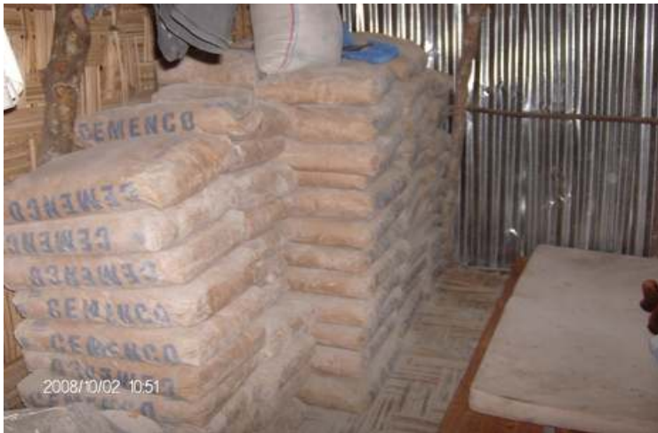
PORTLAND CEMENT STORAGE IN SITE WARE HOUSE.
