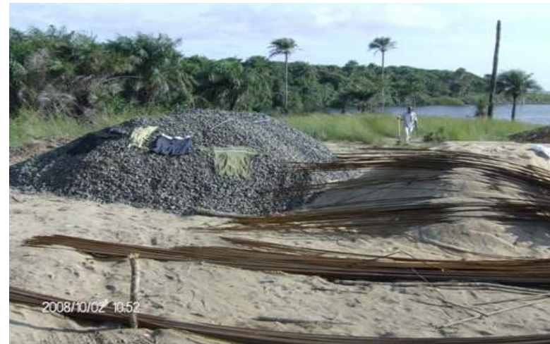
CRUSHED ROCK, BEACH SAND & STEEL REINFORCEMENT BAR DEPOSITS ON SITE.
