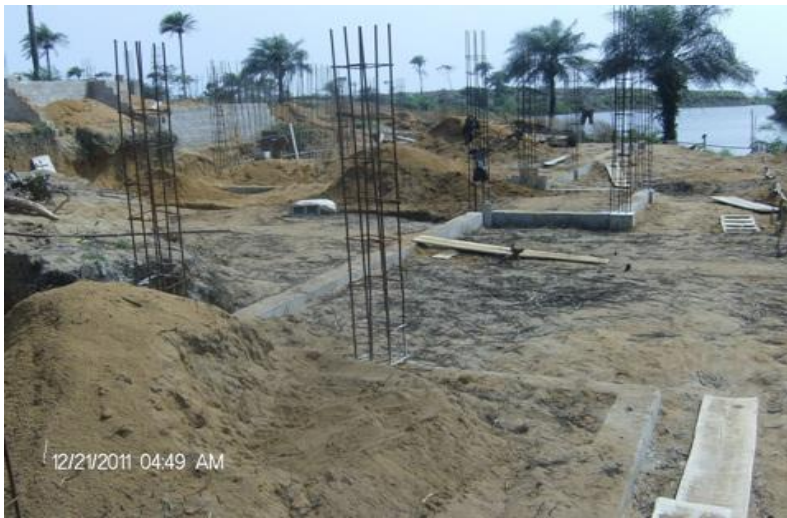
Partial view of basement floor level beyond retaining wall line.
