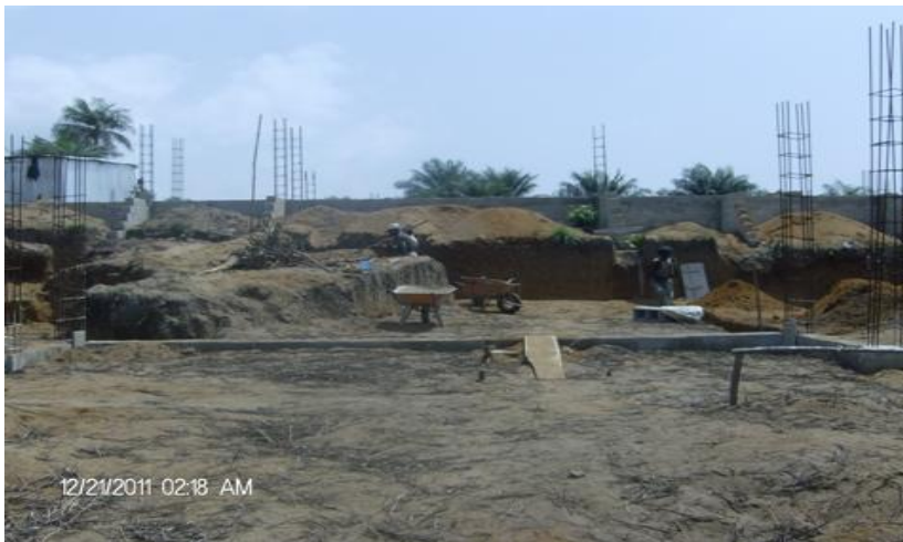
Excavation & clearing to establish basement platform level in progress
