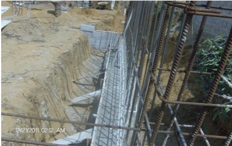
Casting retaining wall footing in progress.
