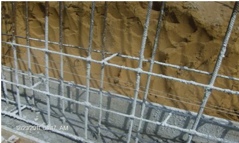
Retaining wall footings showing retaining wall stem steel arrangement.
