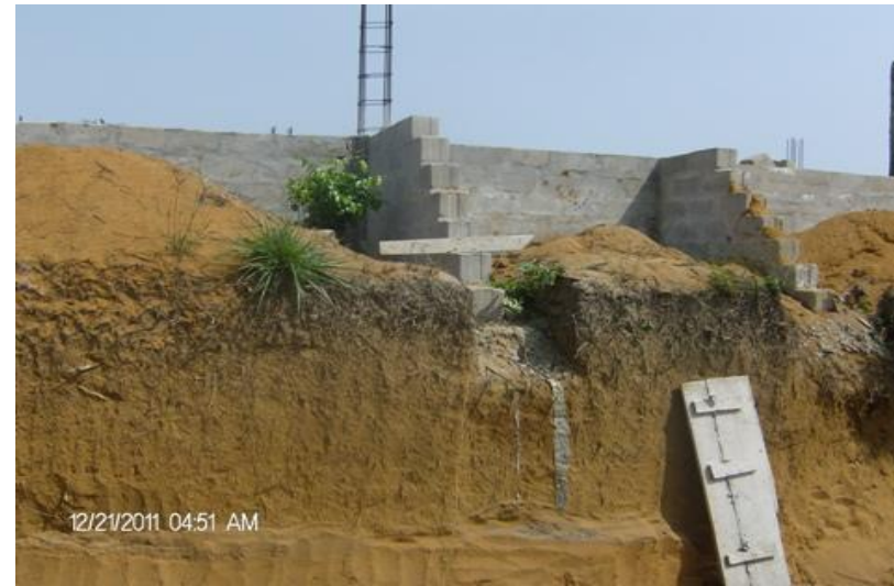
Excavated retaining wall line before installation of retaining wall stem reinforcement.
