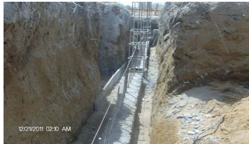
Footing casting for reinforced concrete wall along garage entrance.
