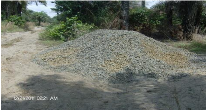
Deposit of crushed granite rocks for construction works.
