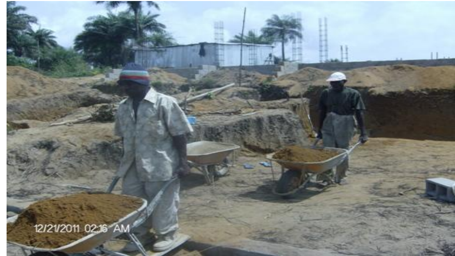
Excavation & clearing to establish basement floor platform level in progress
