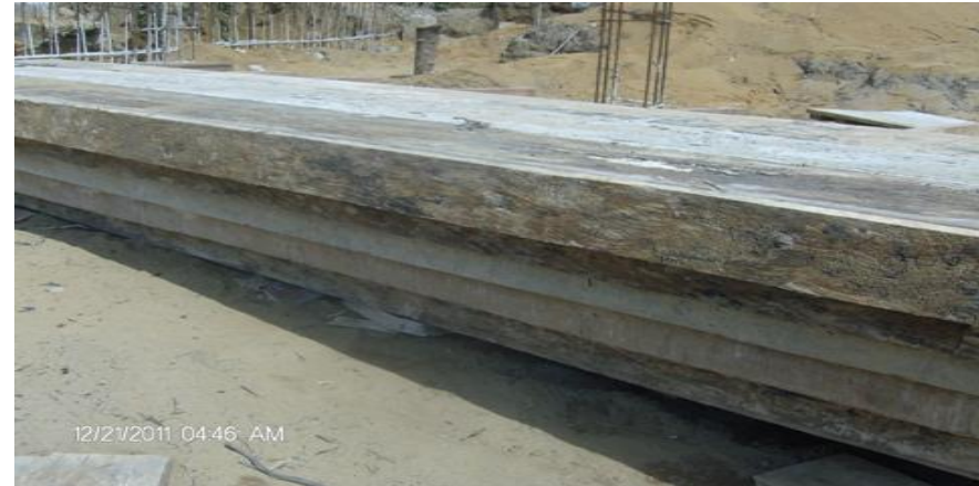
Casting of retaining wall footing within formwork
