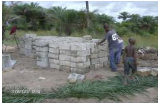
Stock- piling 8" hollow sand- create block for foundation works.
