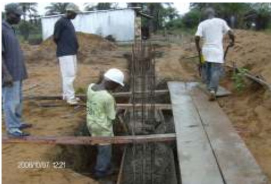
Column footing, dowels & wall footing installation continue
