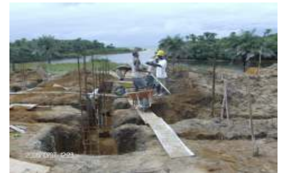
Casting of foundation footings continue
