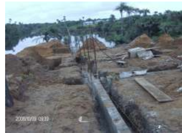
Foundation block wall erection in progress.
