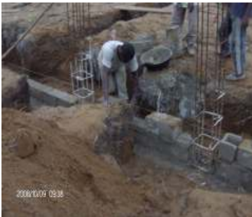
Foundation block wall erection in progress.
