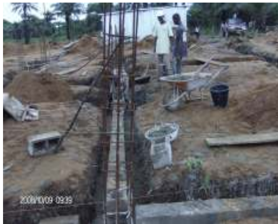
Foundation block wall erection in progress.
