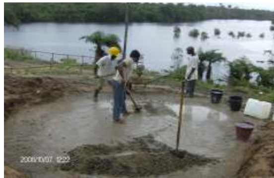
Concrete mixing platform / basin.
