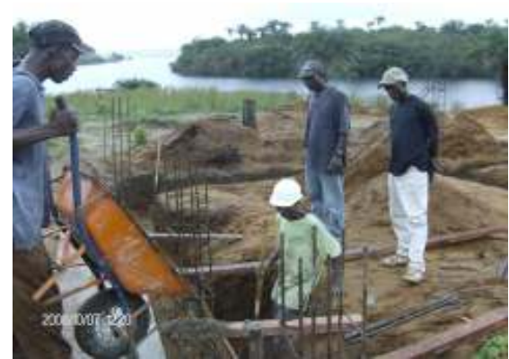
Column footing, dowels & wall footing installation in progress
