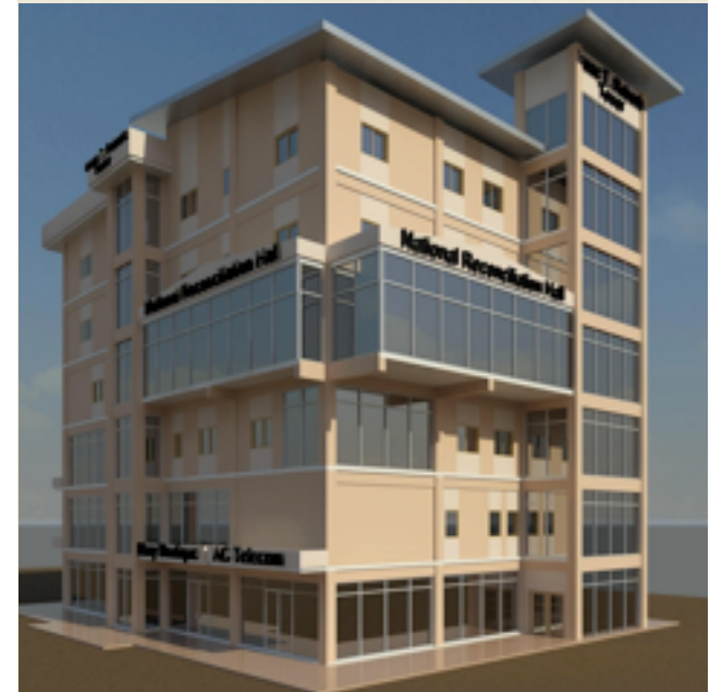
Isaac Togba Roberts Tower @ Red-light
