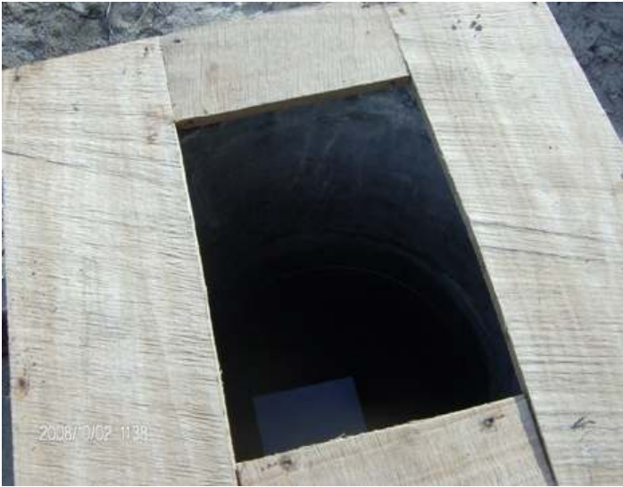
WATER WELL CONSTRUCTED FOR CONSTRUCTION WORKS.
