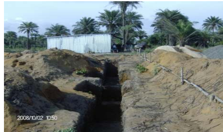
EXCAVATION OF COLUMN & WALL FOOTING TRENCHES.
