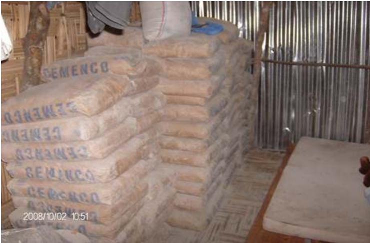
PORTLAND CEMENT STORAGE IN SITE WARE HOUSE.
