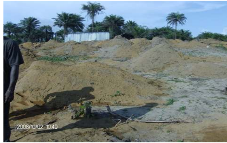
EXCAVATION OF COLUMN & WALL FOOTING TRENCHES.
