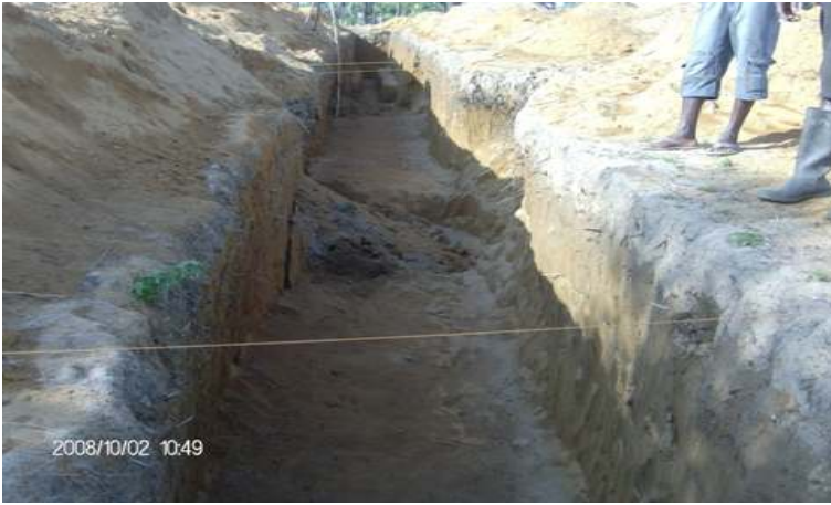
GRID LINE 6 (PROPOSED RETAINING WALL LINE)
