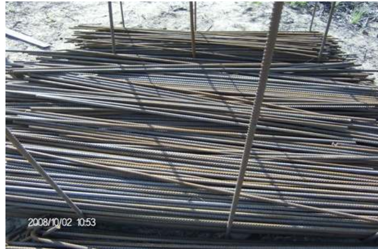
STEEL WORK PREPARATION FOR COLUMN FOOTING MATS & SUB- STRUCTURAL COLUMN DOWELS.
