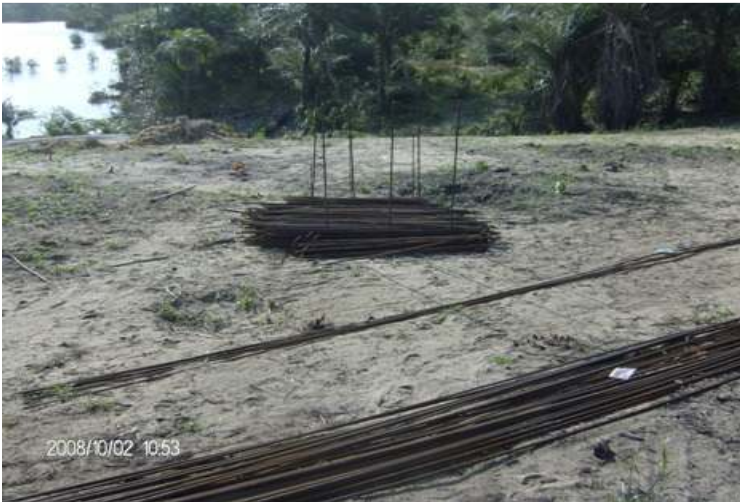
STEEL WORK PREPARATION FOR COLUMN FOOTING MATS & SUB- STRUCTURAL COLUMN DOWELS.
