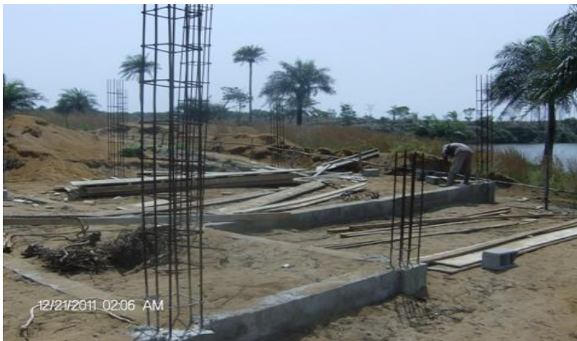
Joinery works for forming of retaining wall stem in progress.
