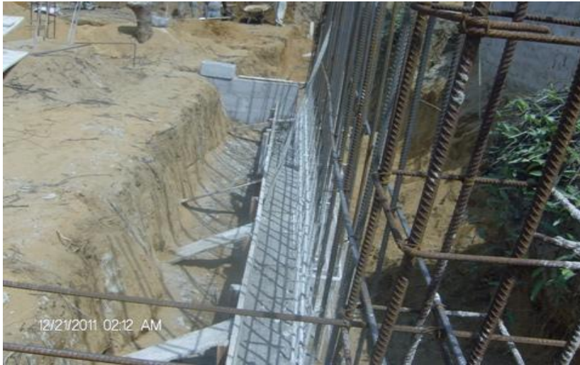
Casting retaining wall footing in progress.
