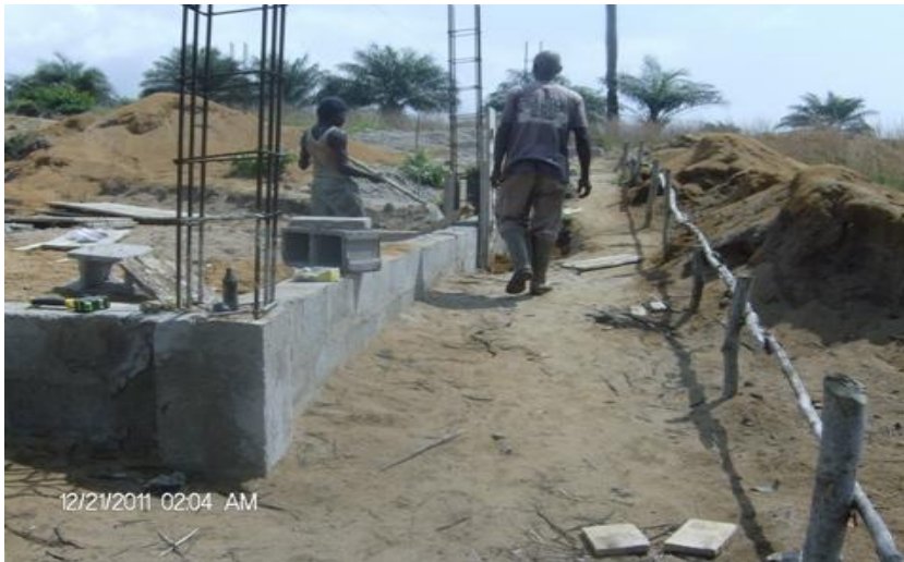
Back filling and spreading of excavated earth material within basement
