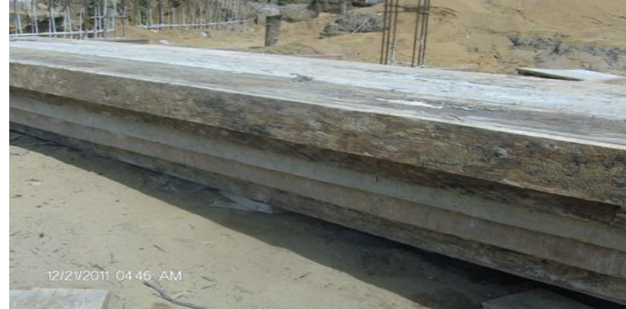
Casting of retaining wall footing within formwork
