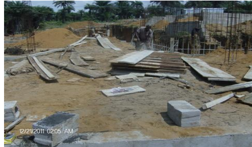
Installation of retaining wall reinforcement & joinery works for forming
