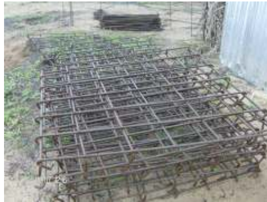
Column footing reinforcement prepared for Installation
