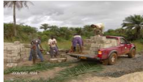
Off- loading blocks for foundation works.
