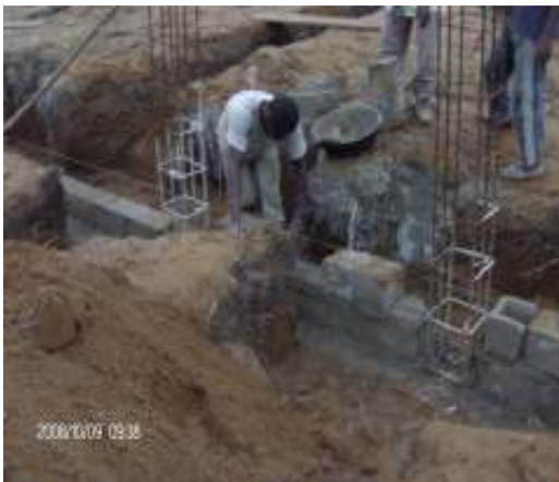
Foundation block wall erection in progress.
