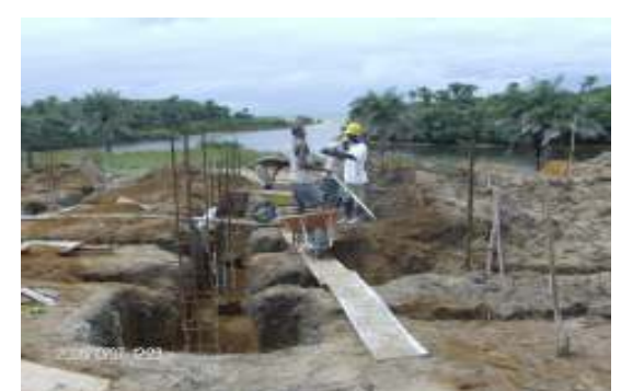
Casting of foundation footings continue
