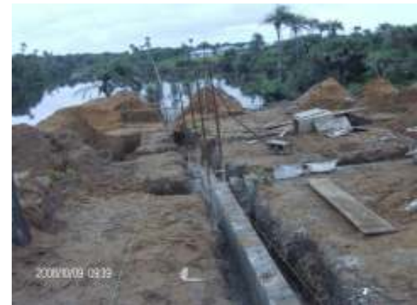
Foundation block wall erection in progress.
