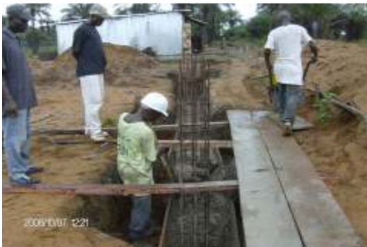
Column footing, dowels & wall footing installation continue
