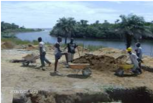
Removal of excavated material within building Envelope.
