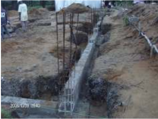
Foundation block wall erection in progress.
