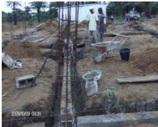
Foundation block wall erection in progress.
